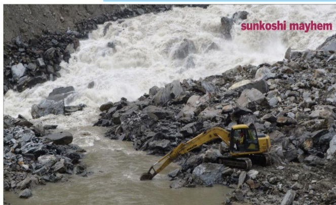
• An excavator at work on Thursday to widen the outlet of a lake that was created on the Sunkoshi river by a massive landslide in Tinjure, Sindhupalchok.
